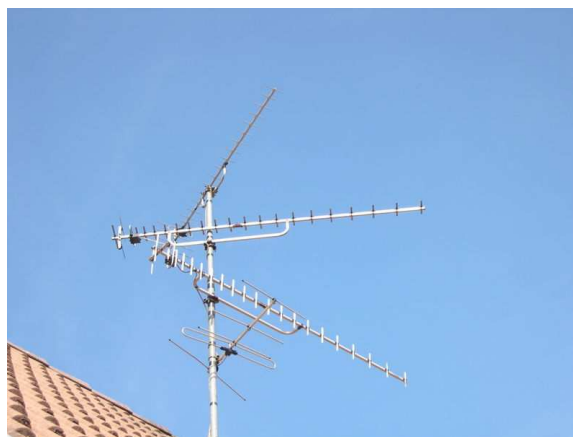
Figure I-5: Antenne Yagi - Uda
