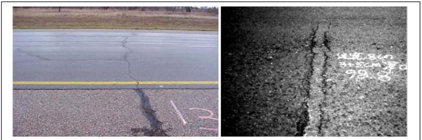
Figure 1.4 – Deux types de fissure réflexive [Zhou 2005]
